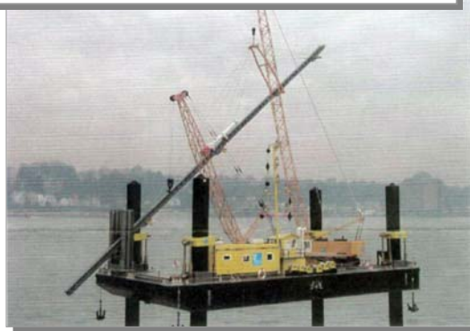
Jack-up working platform "Annegret"
